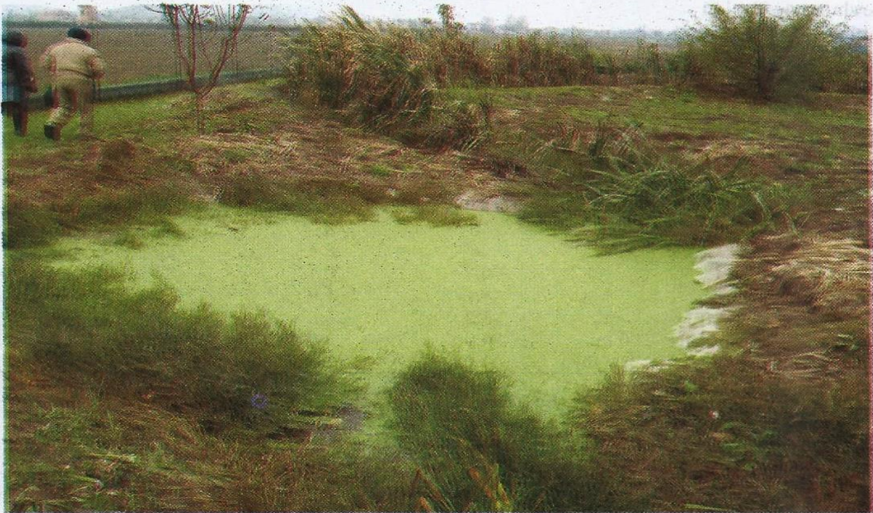
Fig. 9: One of the two aerobic ponds with Lemna spp. growing in it
