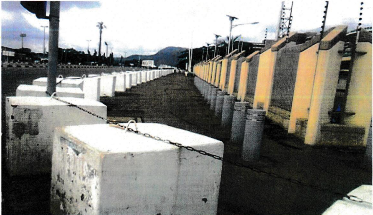
Figure 1: Fixed bollards and Engineered Blocks used as vehicle barrier and also to channel traffic.
