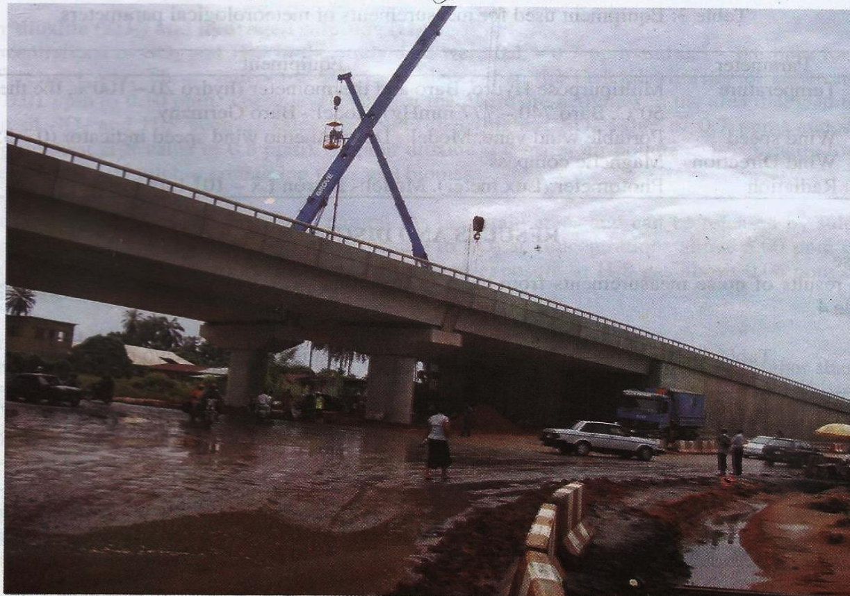
Fig. 4: Itam Flyover Construction site sampling location
