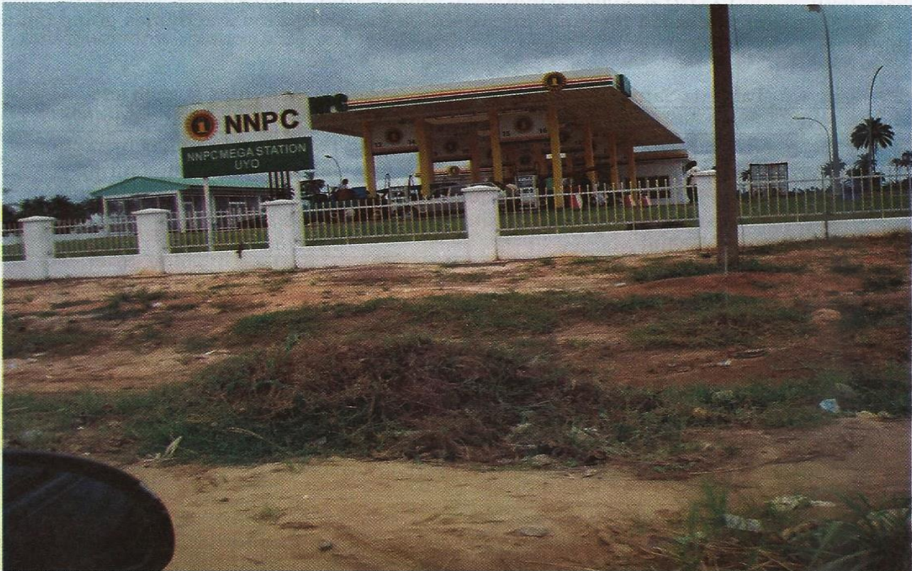
Fig. 2: NNPC Mega Station sampling location
